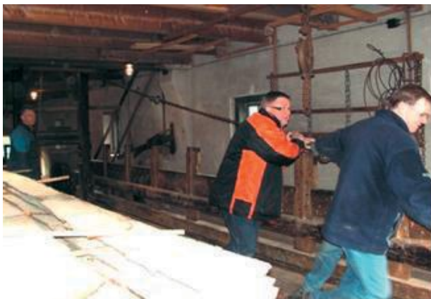
Fig. 15.2.7.1 Running out the cable from the windlass.
