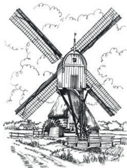
Fig. 17.2.1.2 Wip or hollow post mill (polder mill, some as grain mills).
