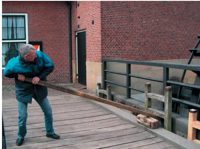
9.4.2.a A timber lever and pivot wood.
